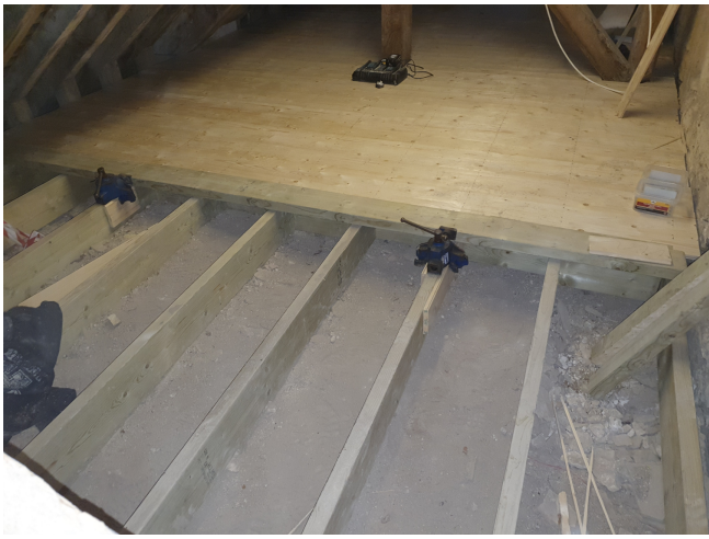
Floor to blower room being installed in the north aisle roof space
