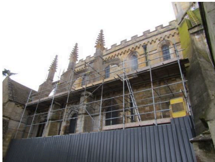
External scaffolding erected on the north side of the Abbey for the removal and subsequent replacement of the north aisle roof tiles after roof felt has been installed.
