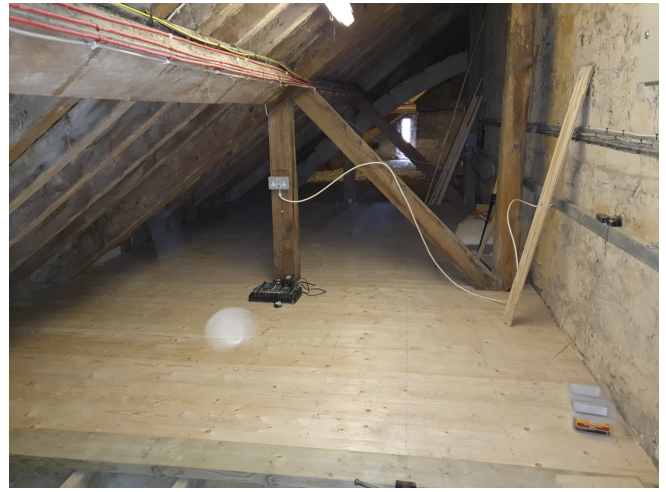
Floor to blower room being installed in the north aisle roof space
